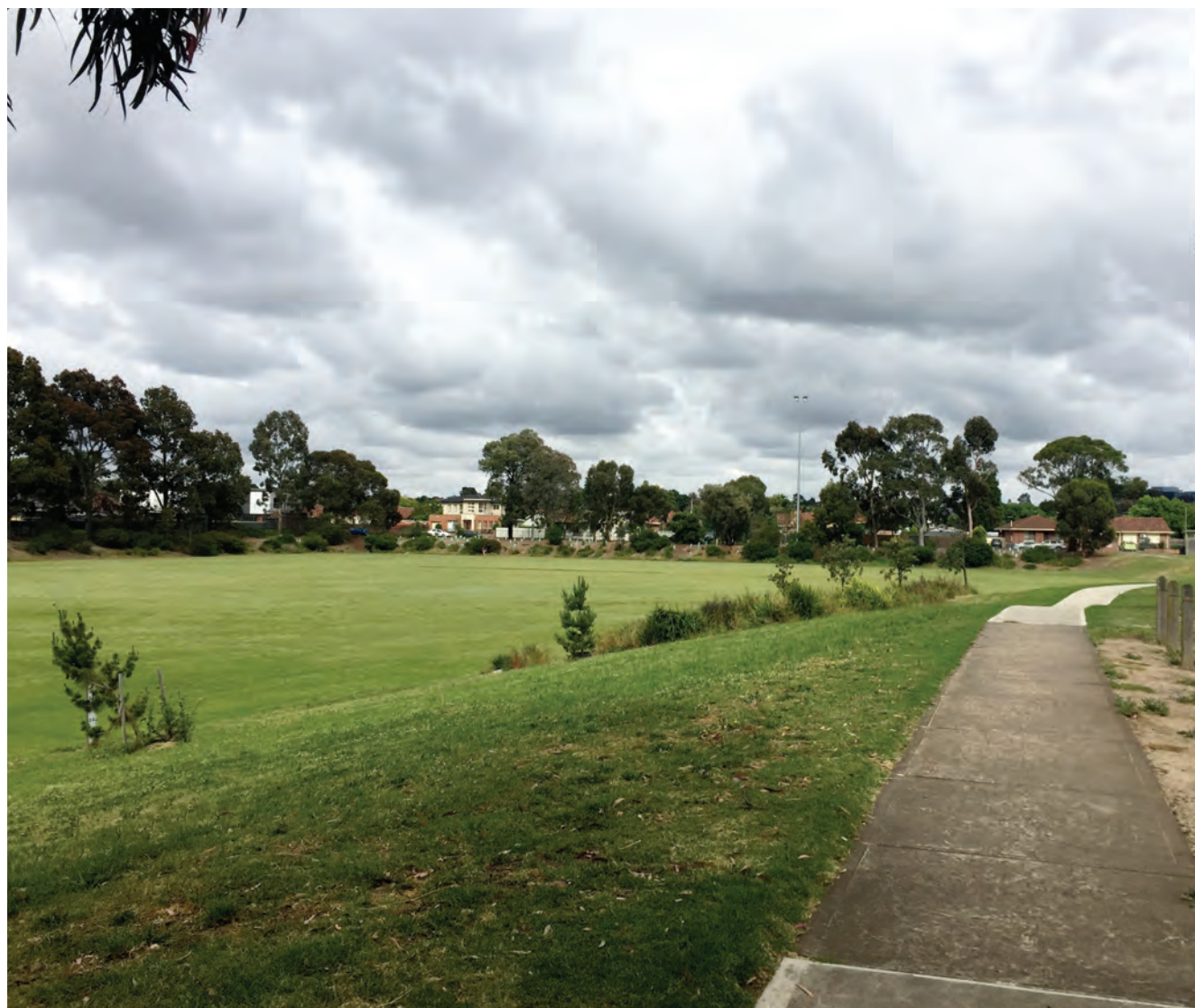
Flood storage basin at HLT Oulton Reserve, Preston where the playing area is inundated in a 20-year flood event but no water enters the basin in any event less than a five-year Average Recurrence Interval (ARI).
