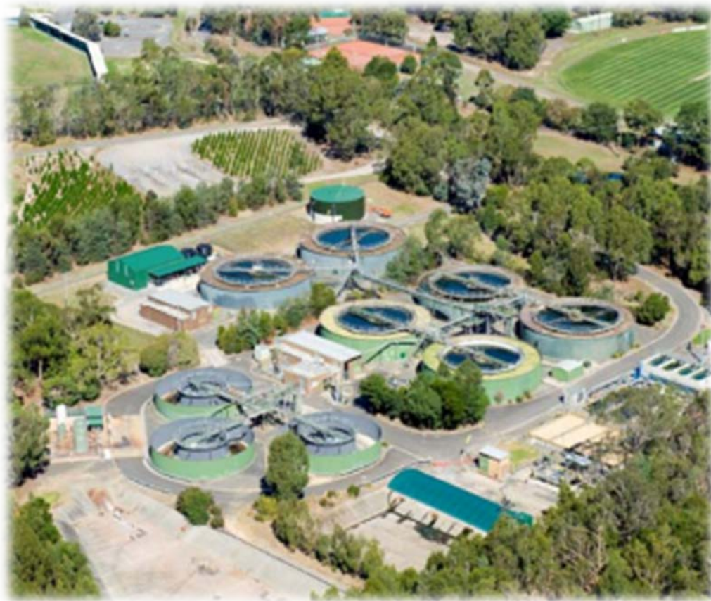
Figure 6: Bushy Creek Treatment Plant
