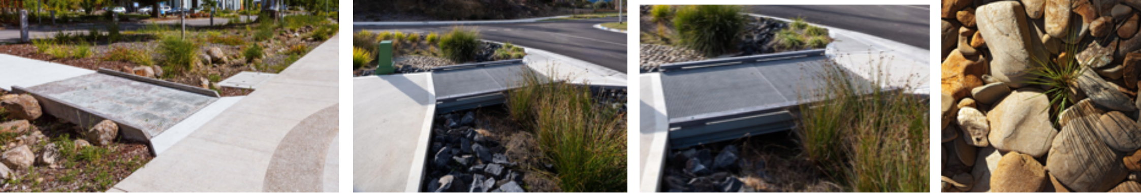
bridges and treatment across vegetated swales
