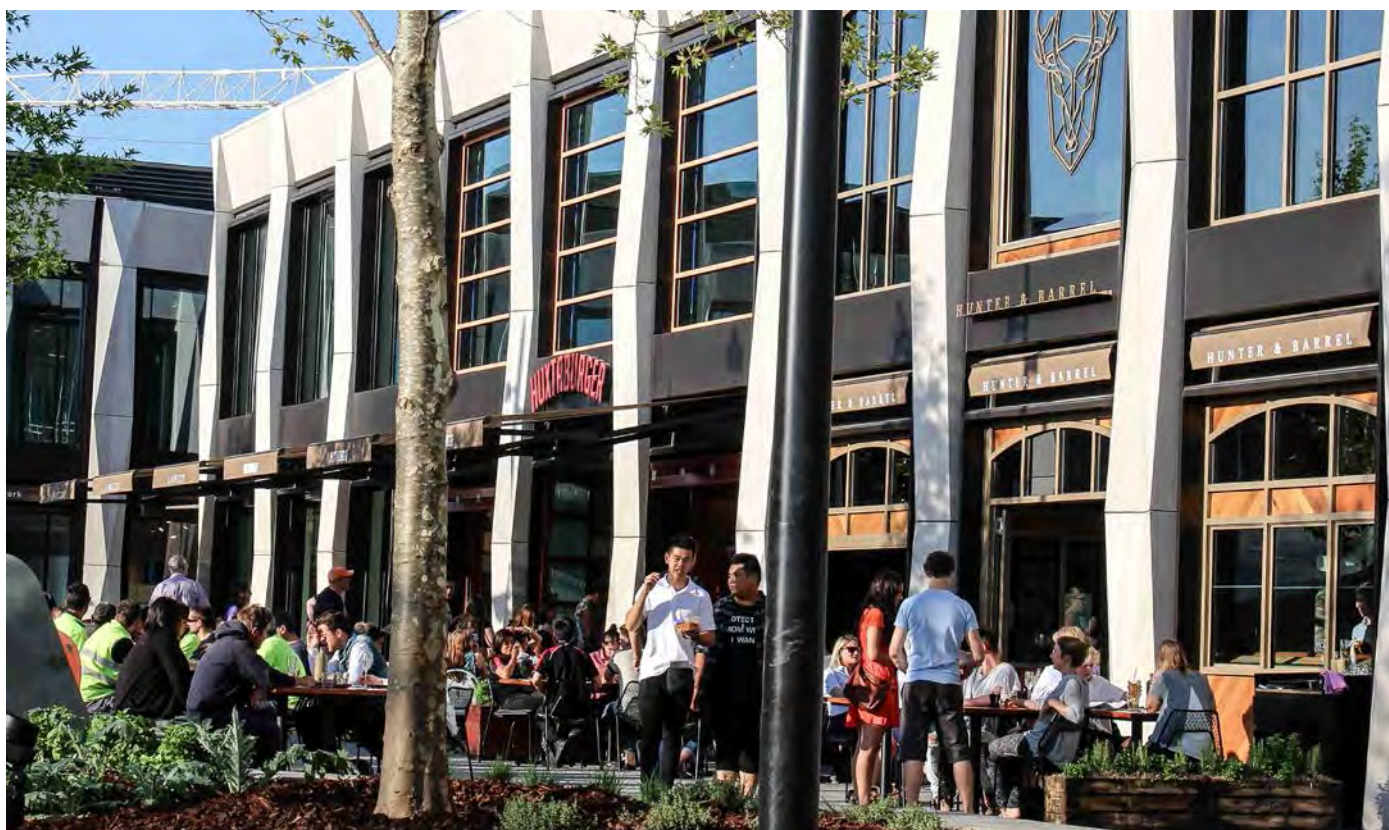
The new Ringwood Town Square in Ringwood was opened as part of the Eastland expansion during 2015
