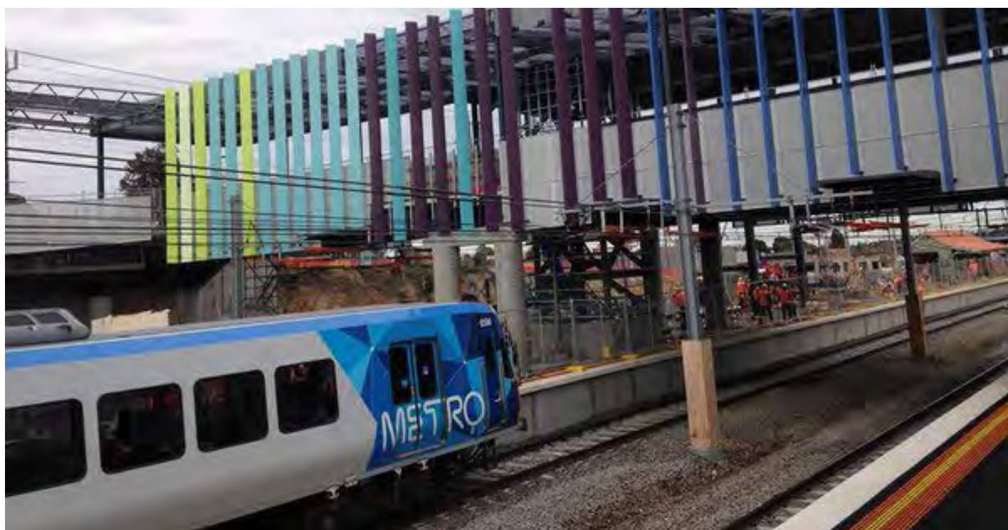
The upgraded Ringwood Railway Station was opened in 2016
