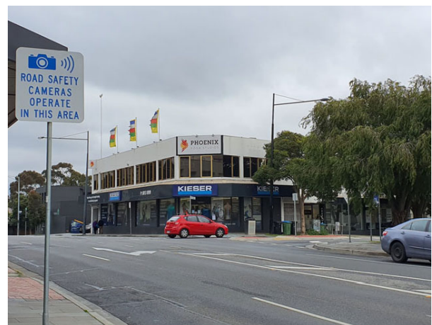
Existing low-rise commercial form on separate land ownership at the corner of Ringwood Street and Seymour Street
