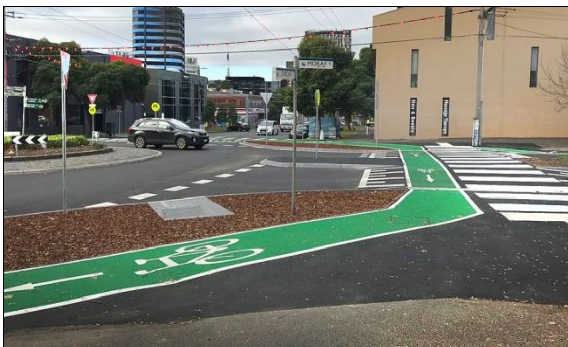
Figure 23 An example of a protected intersection (roundabout) on Moray Street, South Melbourne
