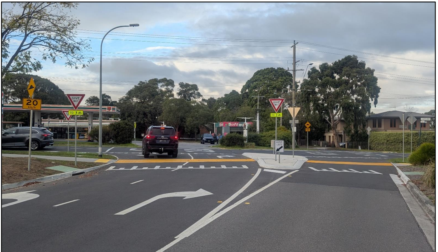
Figure 21 Shared path priority crossing example from Golden Ridge Drive, Corydon Hills
